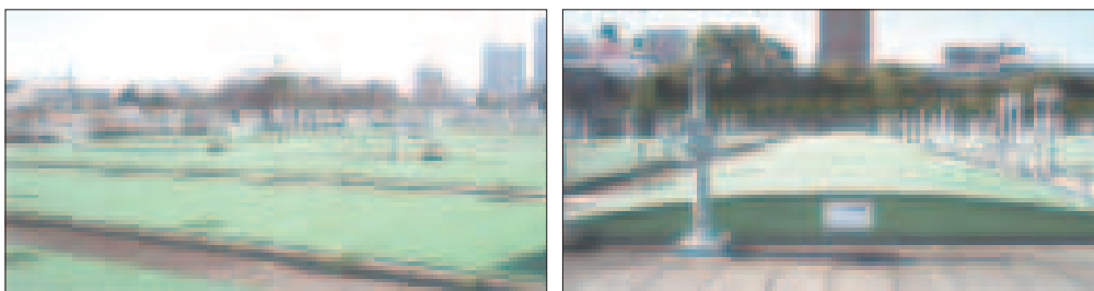
(A) Figure A5.1-1 Covers over sewage structure — Flat type and Dome type (Yokohama City)
